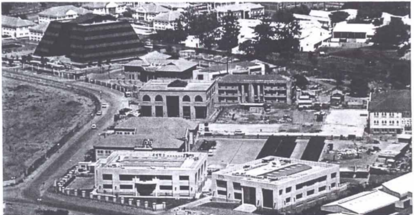
Above: Fairground Area of Gaborone - Tholo Office Park under construction.
