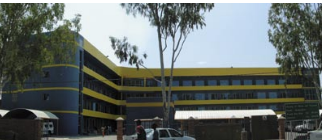
Plaza - now fully refurbished
