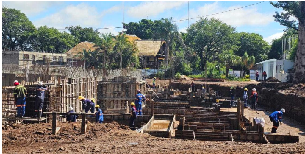
CHOBE MARINA LODGE – REDEVELOPMENT UNDERWAY – FEBRUARY 2026
